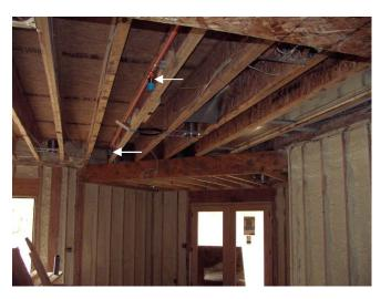
Fire sprinklers being installed in a house under construction on Northview Dr. in Urbandale.
