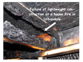
Testing conducted by Underwriters Laboratories shows that structural materials used to build new homes today are prone to collapse sooner when exposed to fire. In addition, homes today are primarily furnished with items made from plastic and synthetic materials which burn faster and release more heat and toxic smoke than furnishings made from natural fibers, significantly reducing the time someone has to escape a fire.
